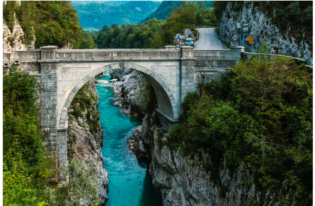
Example of a local alert system installed near a bridge.
